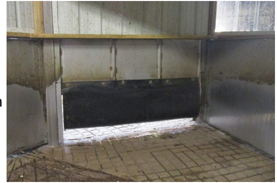
Rubber flap gate ; Vertical slide gates constructed from flexible curtain made from conveyer belting will not injure the pigs if it is accidentally closed on them. Note how the framework that slides in the track is bolted above the curtain.
